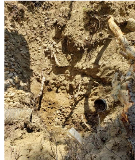
Photo # 2: Close-up of drain discharge.
