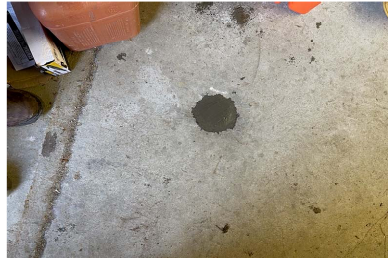
Photo # 4: Floor drain sealed with cement
