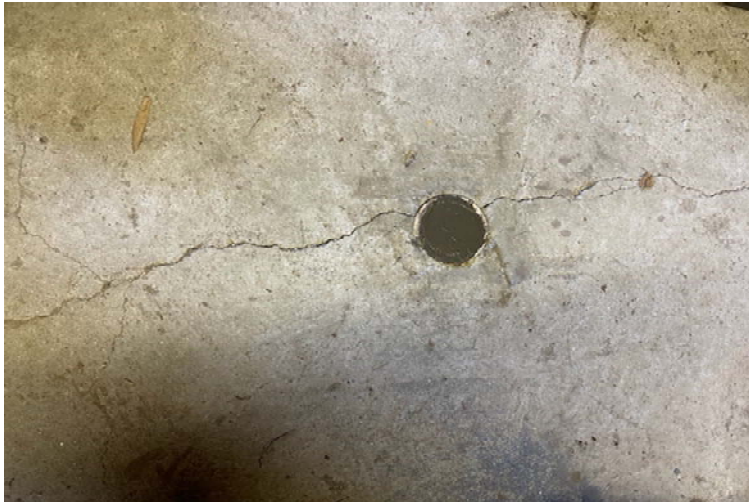
Photo # 3: Floor drain sealed with cement
